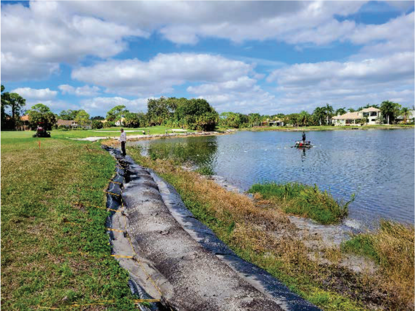
Lower woven B.E.S.T. Tube with "sacrificial" Non-Woven B.E.S.T. Tube
