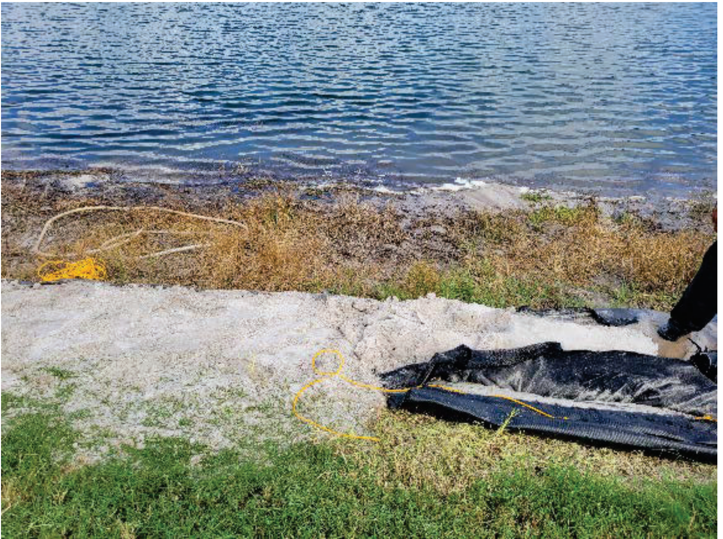
Non-Woven B.E.S.T Tube splayed open prior to hand grading
